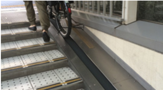
A bicycle escalator in Tokyo (Tamachi Station) © 2014 Stephen-L-Johnson available under CC BY 2.0
