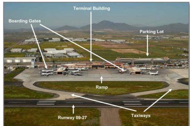
Figure 2.20: Tijuana International Airport
