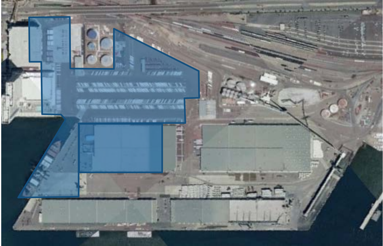
Figure E.22: Tenth Avenue Marine Terminal Facilities
